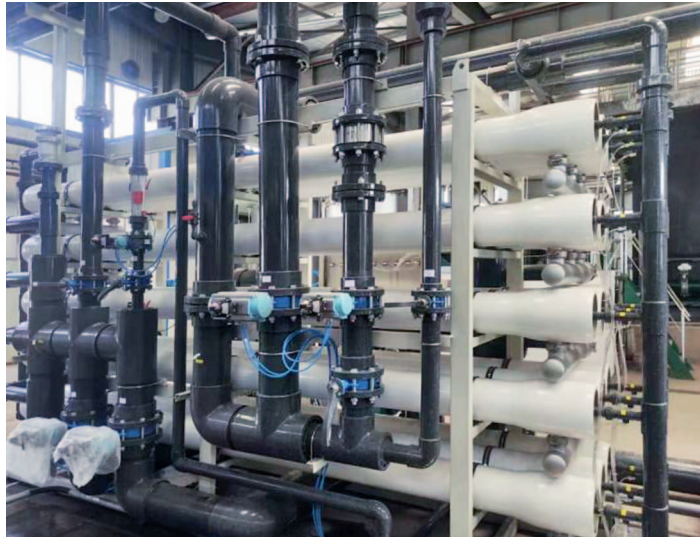
Installed System with Advanced UF Membrane
